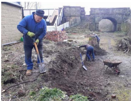
John Holiday digs in to remove mud covering the platform.
